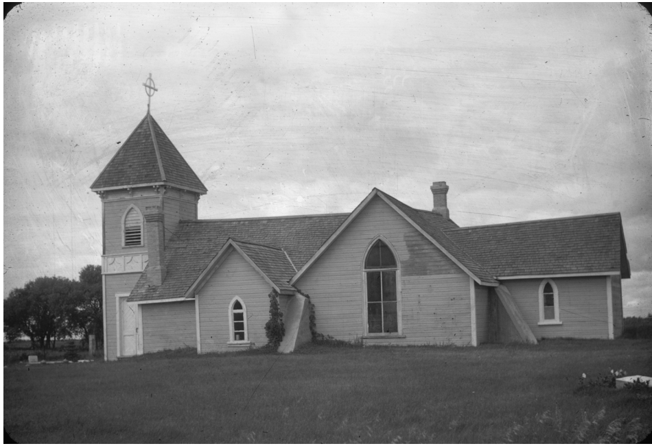
Anglican church built in 1885, Cannington Manor, SK, 5 September 1956. Everett Baker collection.
